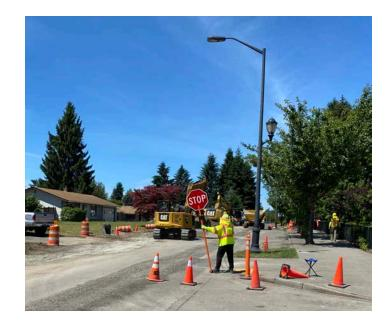
So far just sewer lines are being installed by one crew and the water lines to be installed by another crew. Individual residential hook ups to then follow. Once the main lines are in the City will start the resurfacing of the streets rather than wait for the entire project to be completed. One home owner on 64th Court said that the information was "fantastic" as he was afraid that he would be living with a dirt street in front of his house until next year.
